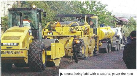
Armenian contractor Chanaparh is now using a Caterpillar RM500 to help recycle roads and provide rapid repairs in Armenia
